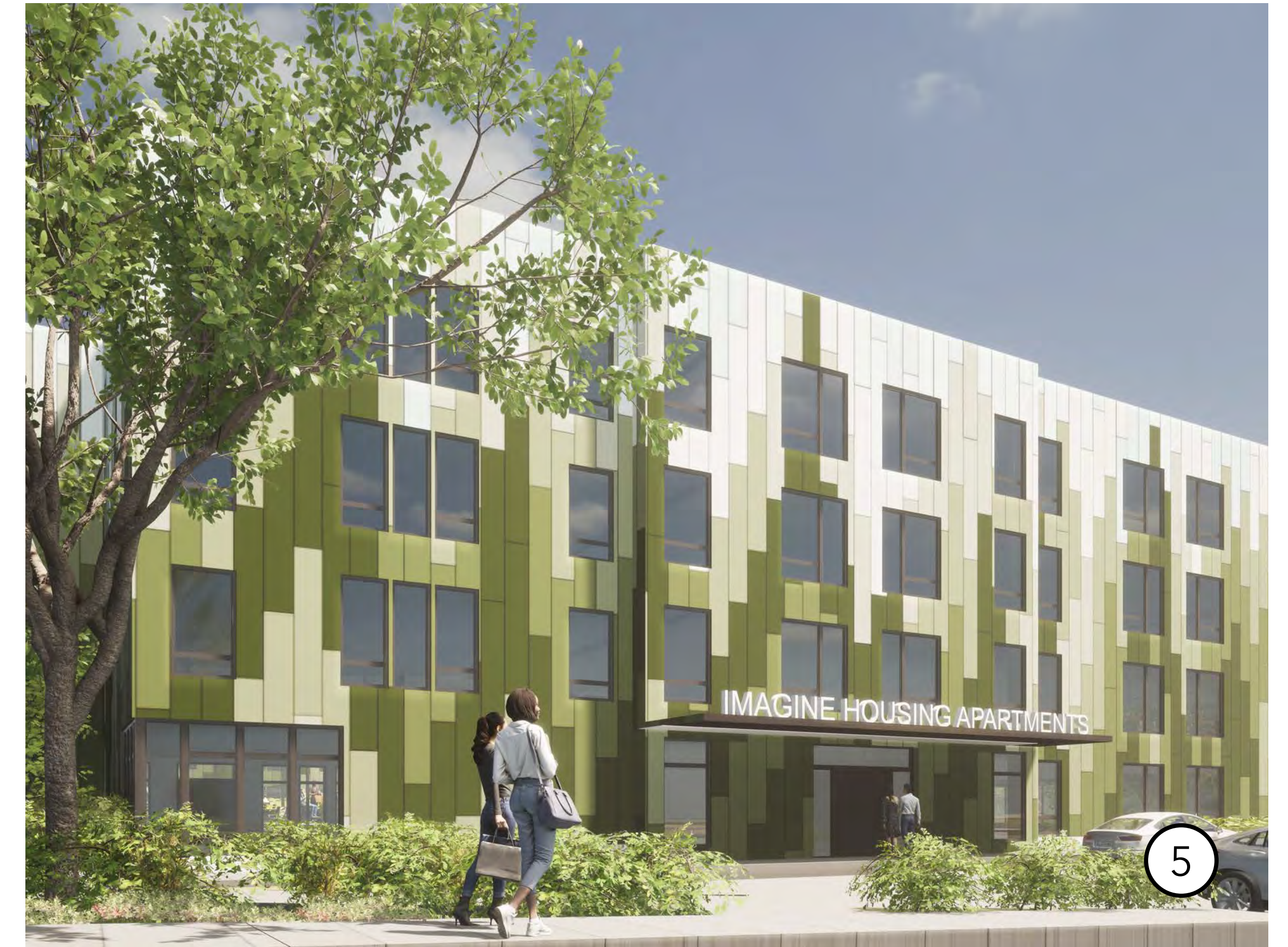
MAIN ENTRANCE TO RESIDENTIAL BUILDING FROM 28TH STREET
